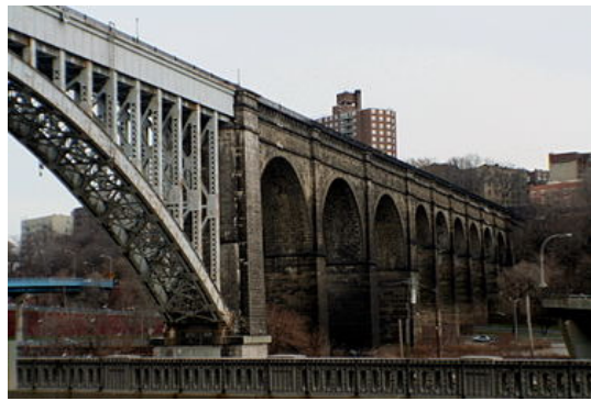
The transition from the steel arch over the Harlem River to the stone arches over the Major Deegan Expressway
